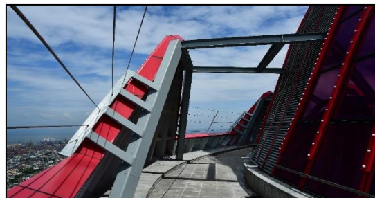
Figure 26: Lotus Tower - Steel structure
