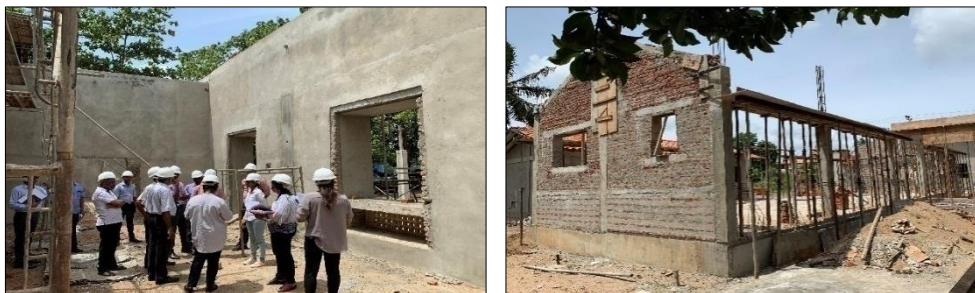
Figure 24: Kadirana Rehabilitation and Renovation Project
